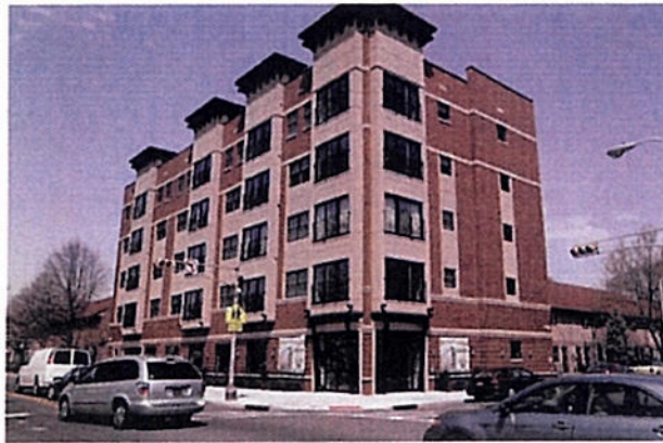
Apartments at Harmony Square, at 105 Broad St., is part of a cluster of projects M&M has created in Newark. "You cannot change a neighborhood with one good building," Maria Elvira Yglesias says. - AARON HOUSTON
